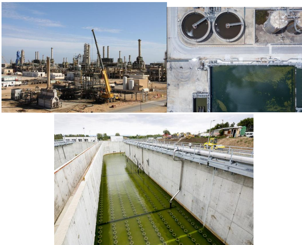
Figure 1 Azzawiya Oil Refinery
