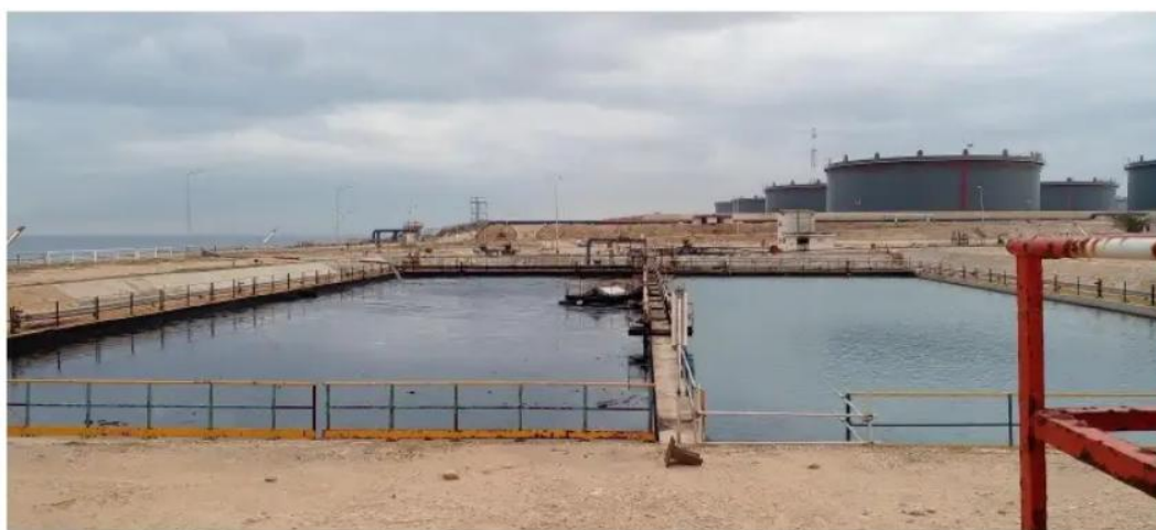
Figure 3 American Petroleum Institute (API) separator at Azzawiya Refinery
